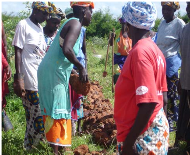
Photo 5: Women building an anti-erosion ring
