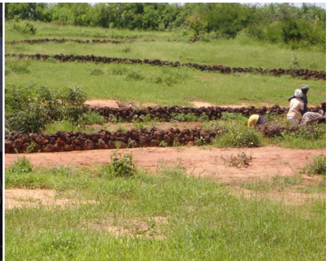
Photo 6: Work in progress
